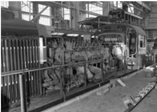
Engine Shop at Syracuse, NY. Servicing ALCo/GE RS-3 at DeWitt. (NYCSHS Collection)
