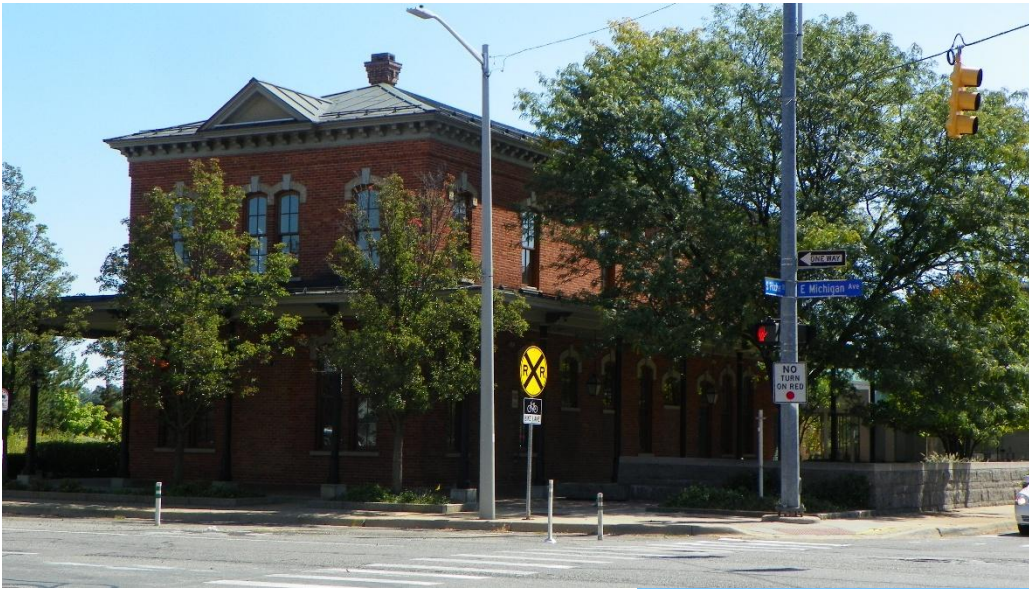
Kalamazoo (above and right) Grand Rapids & Indiana (PRR) Passenger with separate freight house 406 E Michigan, Kalamazoo GPS 42.292912, -85.578617 Kalamazoo Community Foundation
