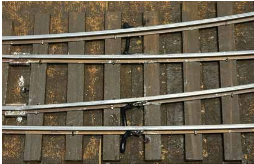
Jumper wires between stock rails and closure rails.
