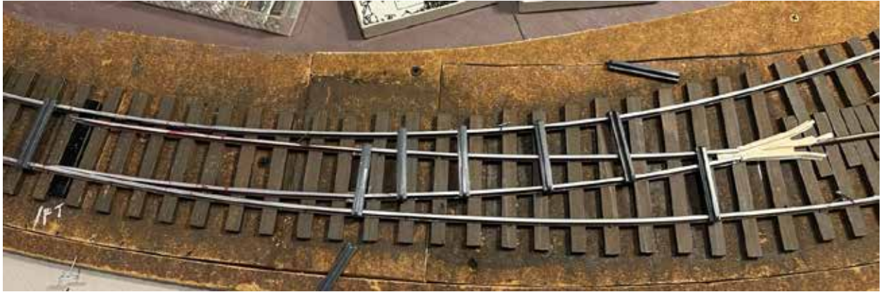
Preliminary fitting before spiking closure rail associated with lower rail.
