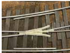
Guard rails in place.
