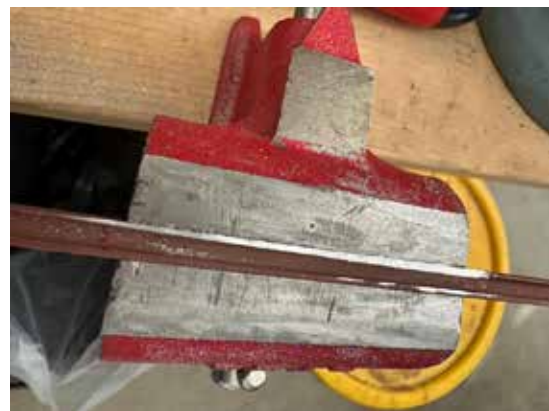
Stock rail base flange being filed.
