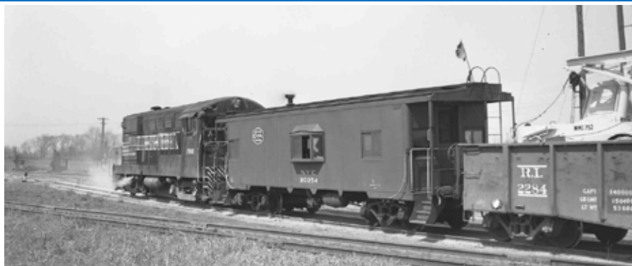
NYC H-20-44 7111 pushing 69 cars on East Hill where all switching was done on a considerable grade and required a yard locomotive with lots of guts. NYCSHS Collection
