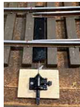
Ground throw installed.
