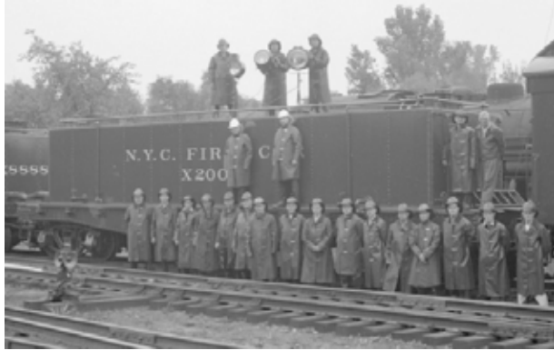
The rivet details can clearly be seen on this original photo of the fire car. NYCSHS photo collection.
