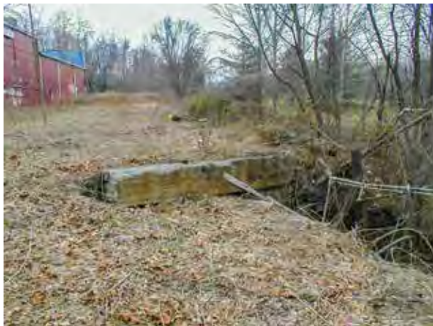
The concrete support to start the track rise for the coal facility.
